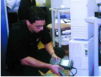
spikes and line interference are generated, the full time isolating power conditioned UPS absorbs these potentially destructive transients — protecting the store's systems. The UPS also re-establishes the neutral-ground relationship to enhance the electrical environment and improve equipment performance — eliminating “lock-ups” and operating errors. The UPS is also capable of delivering
